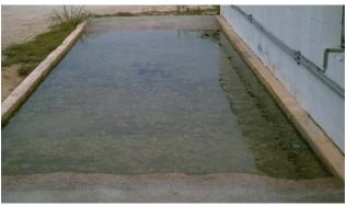
Note lack of a sump, or slope. Collecting a spill would be difficult.
