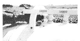
VALVES must be clearly labeled or color coded: Orange/Red for liquid and Yellow for vapor.
